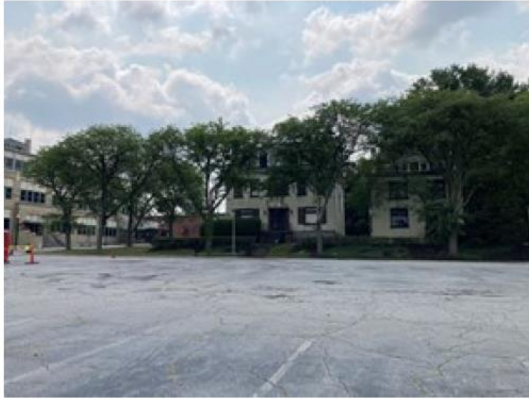
Image one: Paved parking lot located at the front of 7228-7930 McPherson Blvd
