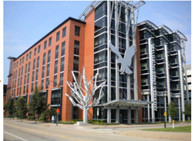
American Eagle Outfitters Headquarters
