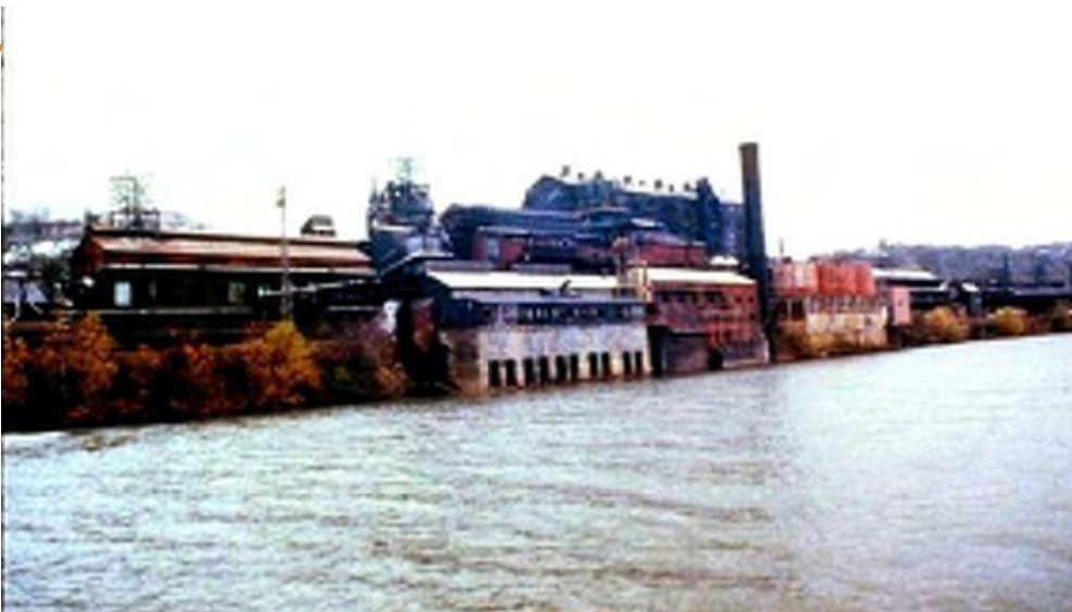
Solid river walls provided the opportunity for creative on-site engineering
