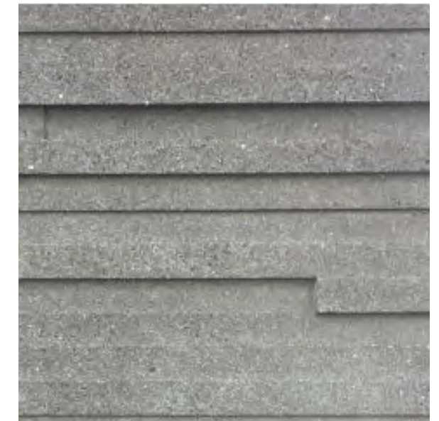
Accent Concrete Walls- Board Form Finish
