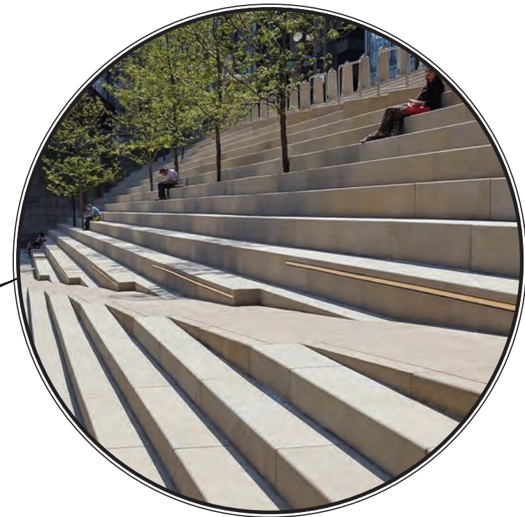
integrated steps and sloped accessible walkway
