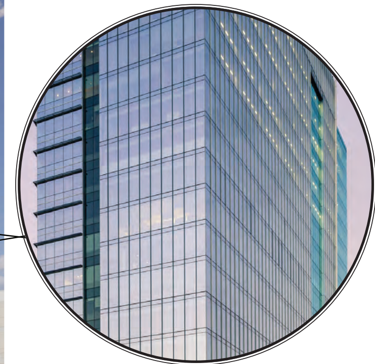
curtainwall with mullion "fin" extensions
