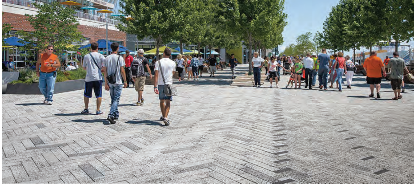
Plank Unit Paving (mix of grays/paver finishes)
