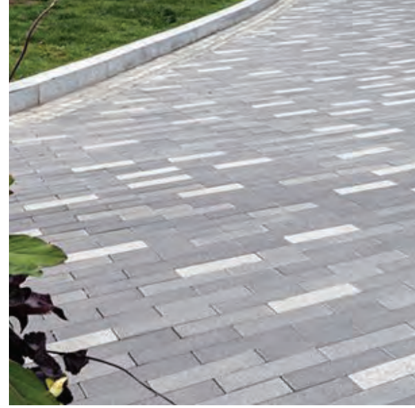
Plank Unit Paving
