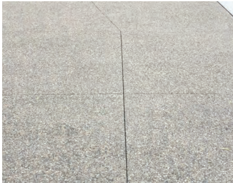
Exposed Aggregate Concrete (ROW sidewalks-accent)
