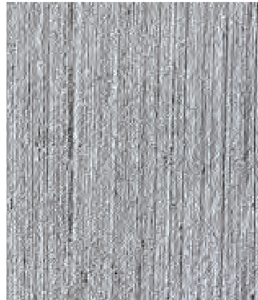
Broom Finish Concrete
